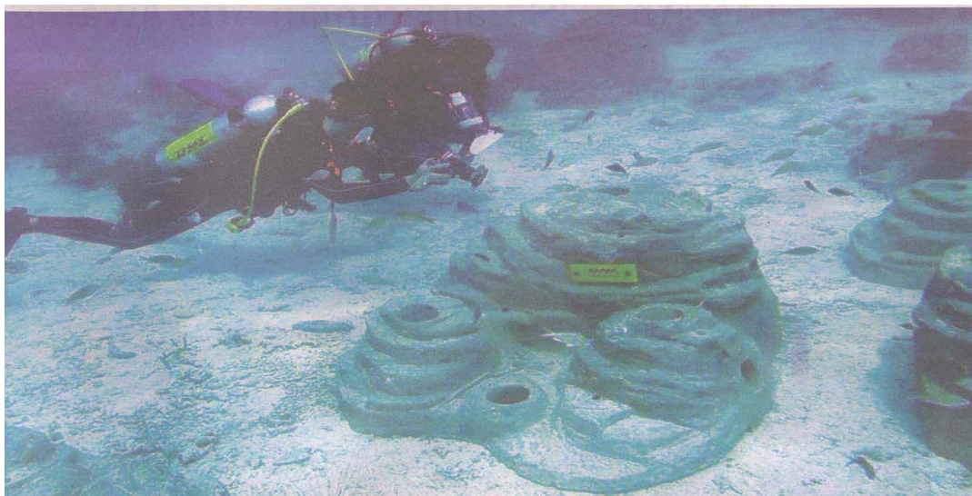
Divers checking out a newly placed Aquascape artificial reef. Each unit of the cement mound weighs 400kg and is designed to resemble natural seascape. — Picture by Trinna
